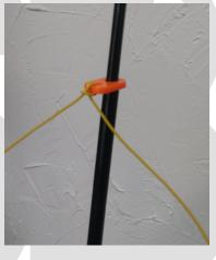
This gives you a firm attachment point which will slide onto a telescopic pole or that you can tie a cord to. Alternatively you could use a handy tree-branch to support this part of the aerial. Aim to get the attachment point of the aerial at least 4 metres (13 ft) up in the air.
